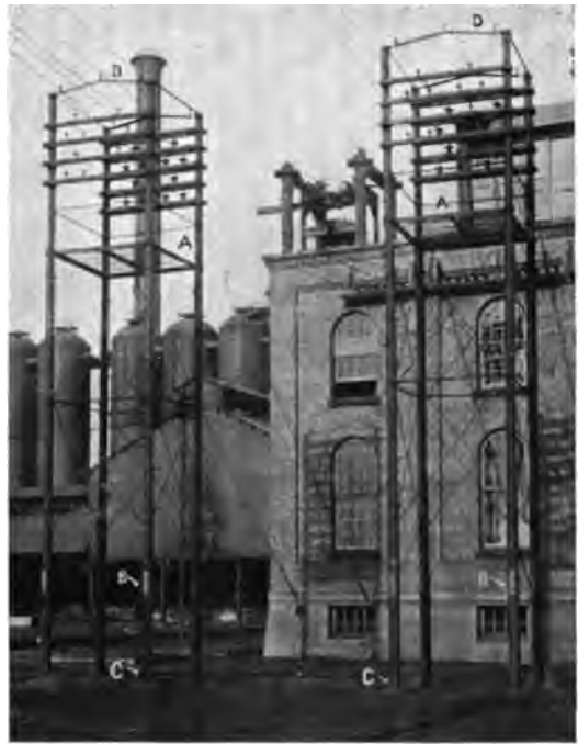
Fig. 2. High-Tension Towers. (National Tube Company.)
